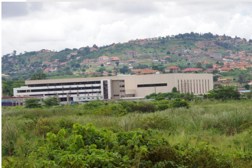
The recently constructed NMS warehouse in Kajjansi, off Entebbe Road.
